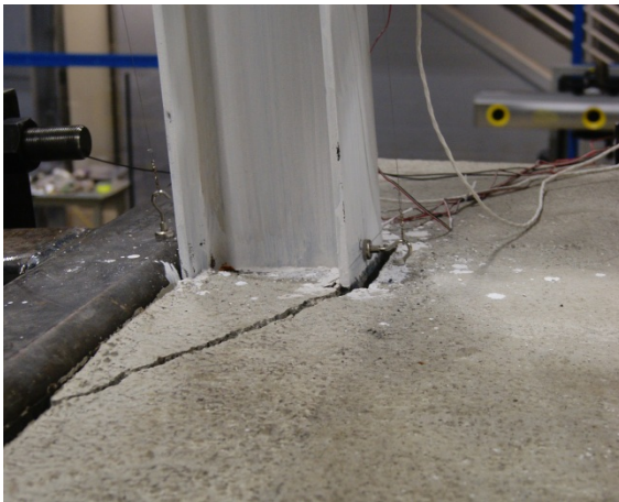
(a) North view of concrete slab around east column
