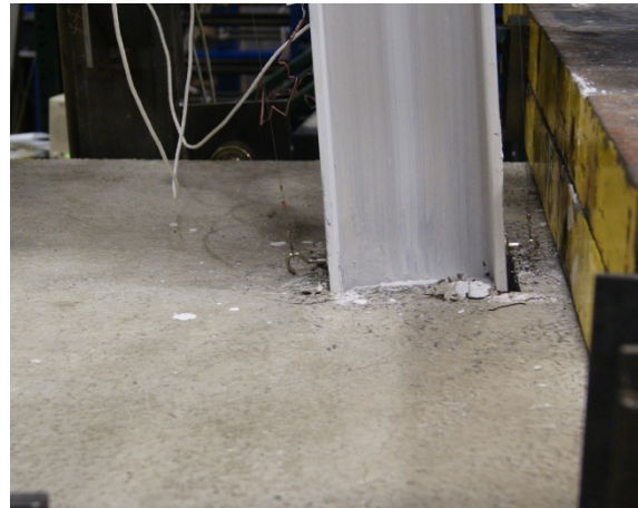
(b) North view of concrete slab around west column
