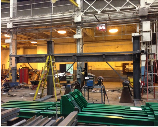
(a) Overview of specimen at construction site
