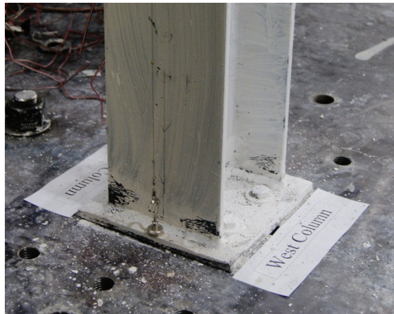
(d) East-north view of west column; HS02-160%
