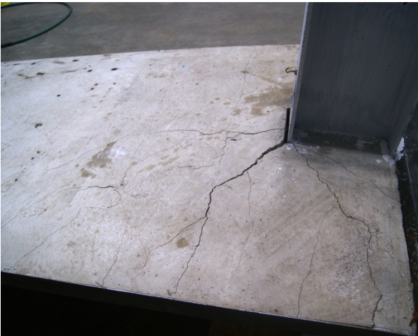
(b) South view of concrete slab at east column
