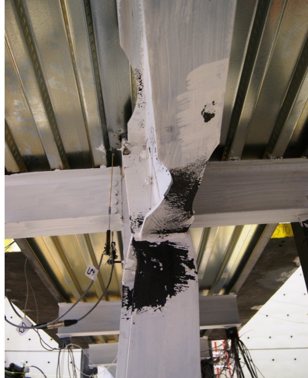
(b) Girder with RBS at west joint [-0.078 rad.]
