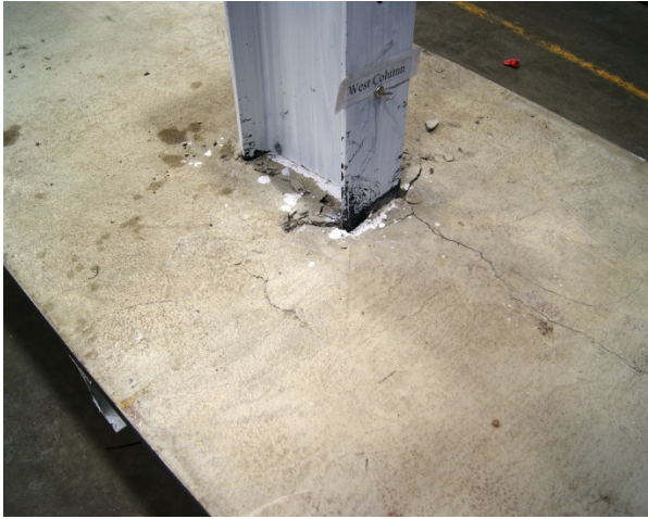
(c) North-west view of concrete slab at west column
