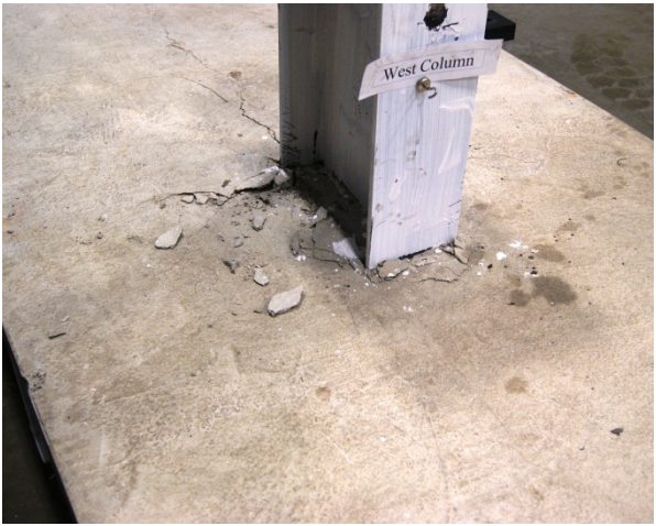
(d) South-east view of concrete slab at west column
