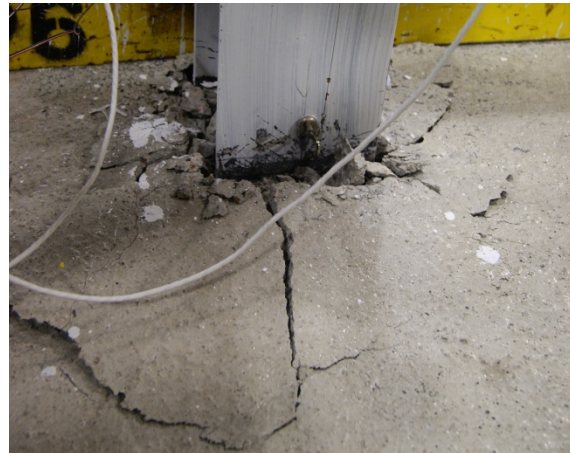
(b) East view of slab around west column
