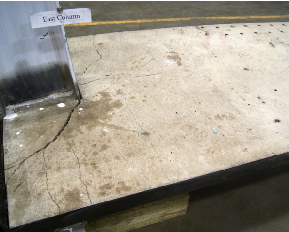
(a) North view of concrete slab at east column
