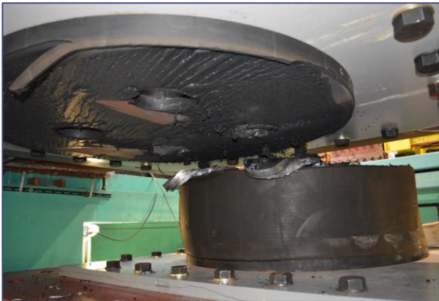
Rupture due to delamination
